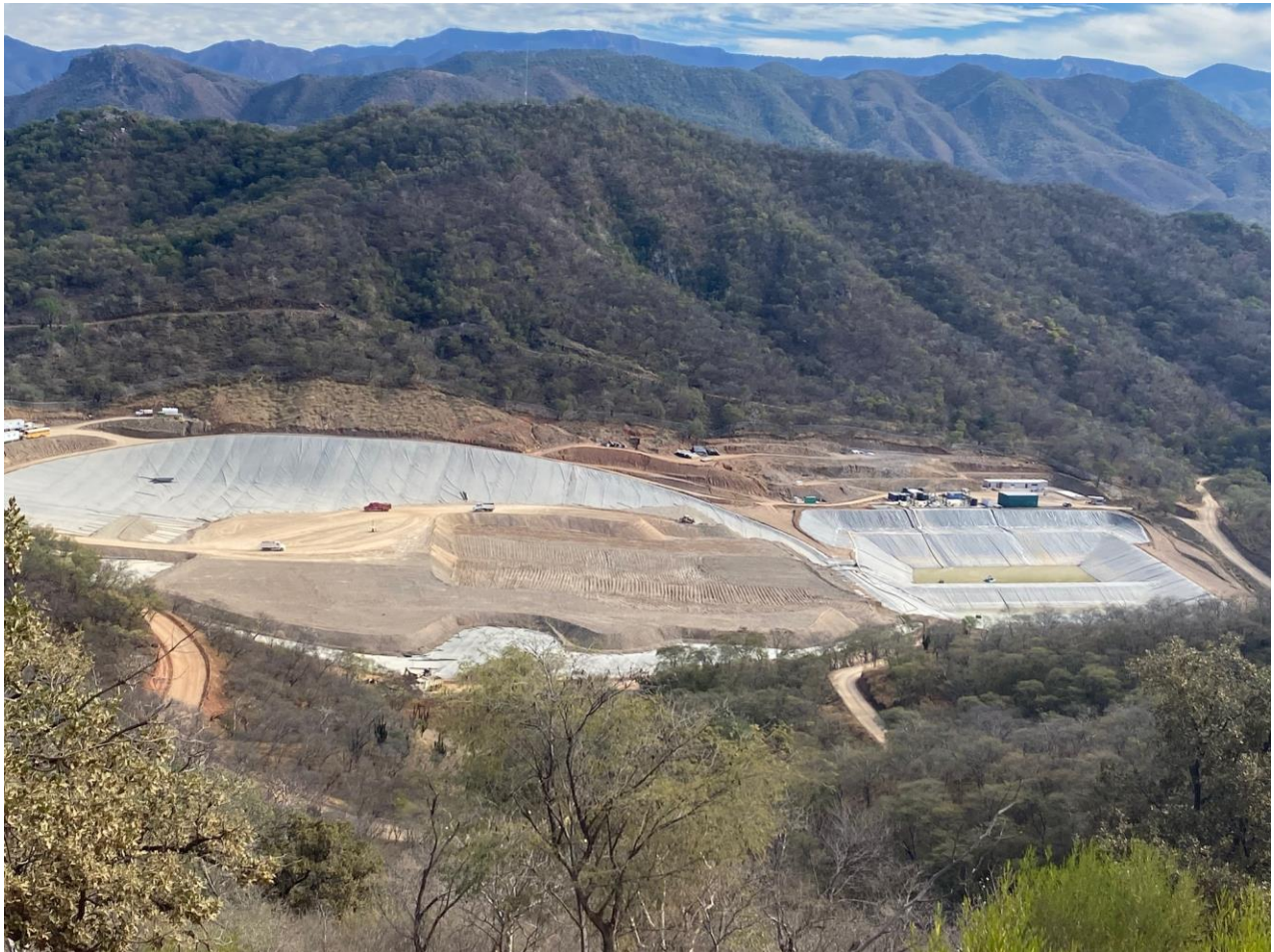
Photo 1: Advancement of stacking and leaching activities at Santana heap leach pad
