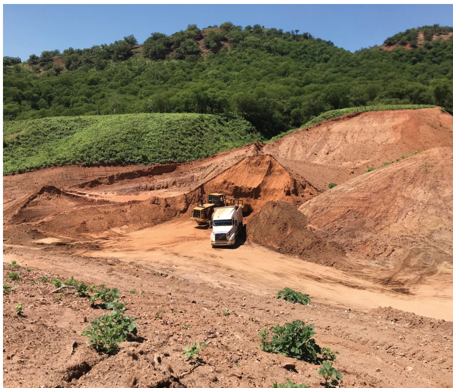
Ongoing earthworks during pad construction at Santana
