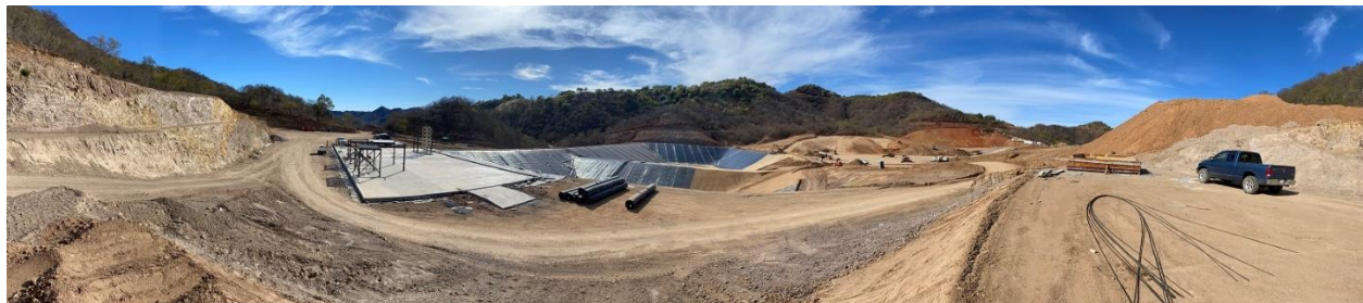
Photo 2 – Panoramic Site showing Plant foundations adjacent to Solution Ponds (December 2020)
