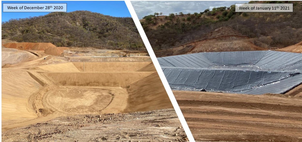
Photo 1– Lined Solution Ponds with Plant location in background
