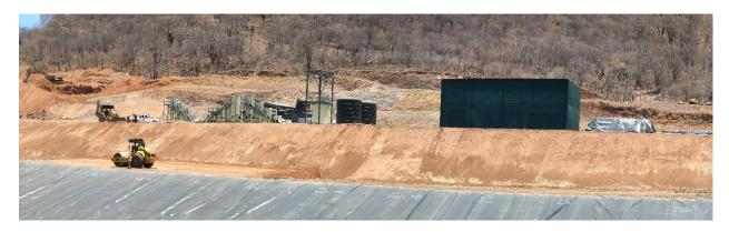
Photo 3 - Gold recovery (carbon) plant completed and awaiting start of commissioning
