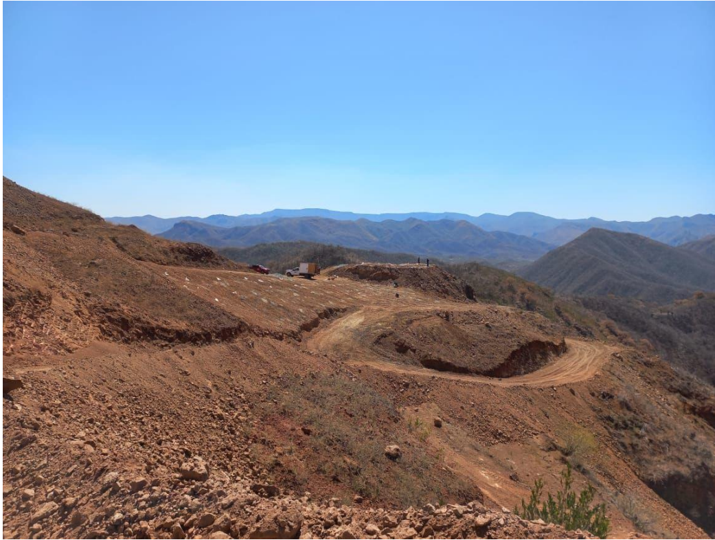
Photo 2 - May 13 th , 2024 – Blasting set up for establishment of future bench development
