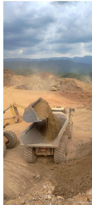
A series of photos highlighting the progress being made in August 2024 at the new Nicho Main zone pit development
